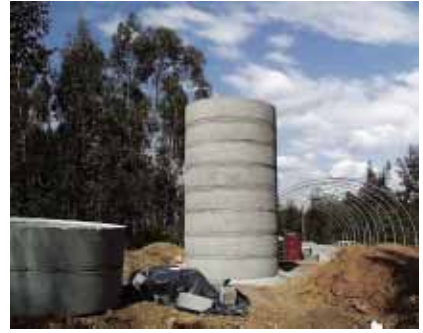
Water tank being built for irrigation. All gravity flow.
